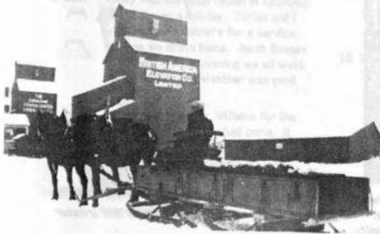
This picture, courtesy Mrs. Klaas Kroeker, shows how coffins were brought to the church in the early days. The elevators have an important role in the Schmidt family. The first one was where Uncle John was agent, i. e. B. A. Elevator. The Canadian Elevator was where Uncle Aron was agent. The third one, behind the Canadian, was the U. G. G. where my father was grain buyer. They were buyers at different times.
